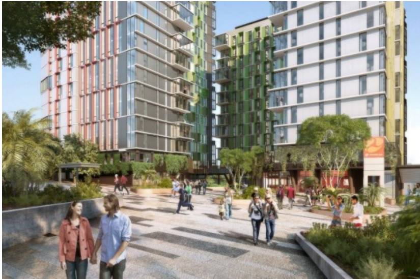
Interger is developing the 1578-bed Unilodge facility at Buranda in Brisbane. Supplied
